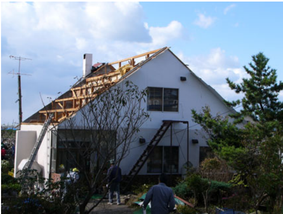
図 9 屋根葺き材の飛散(A damaged house whose roof materials were peeled off)
