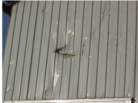
図 12 外壁への飛来物の衝突(A trace of windborne missile on a wall of wooden house)
